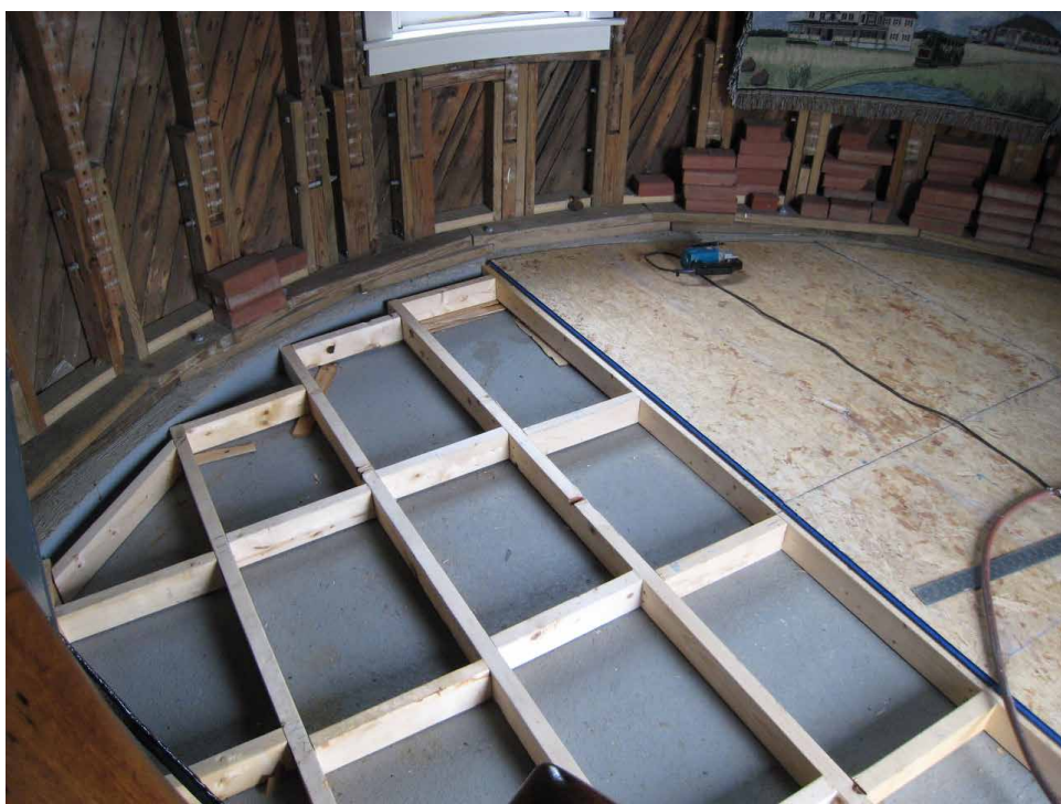
Replacement of lighthouse floor
