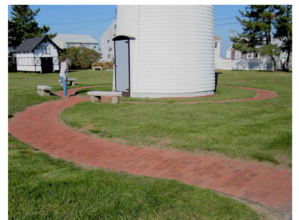
Installation of brick
