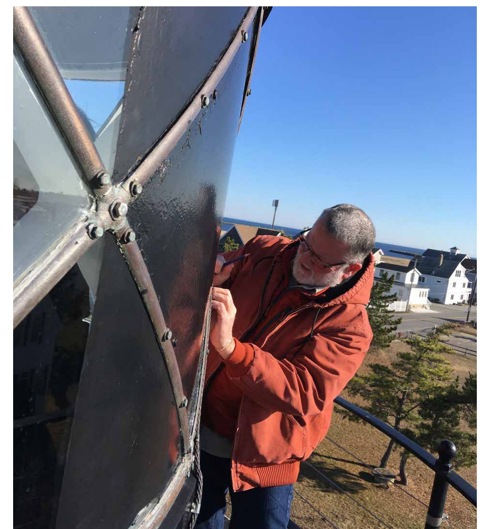
Installation of replacement glass
