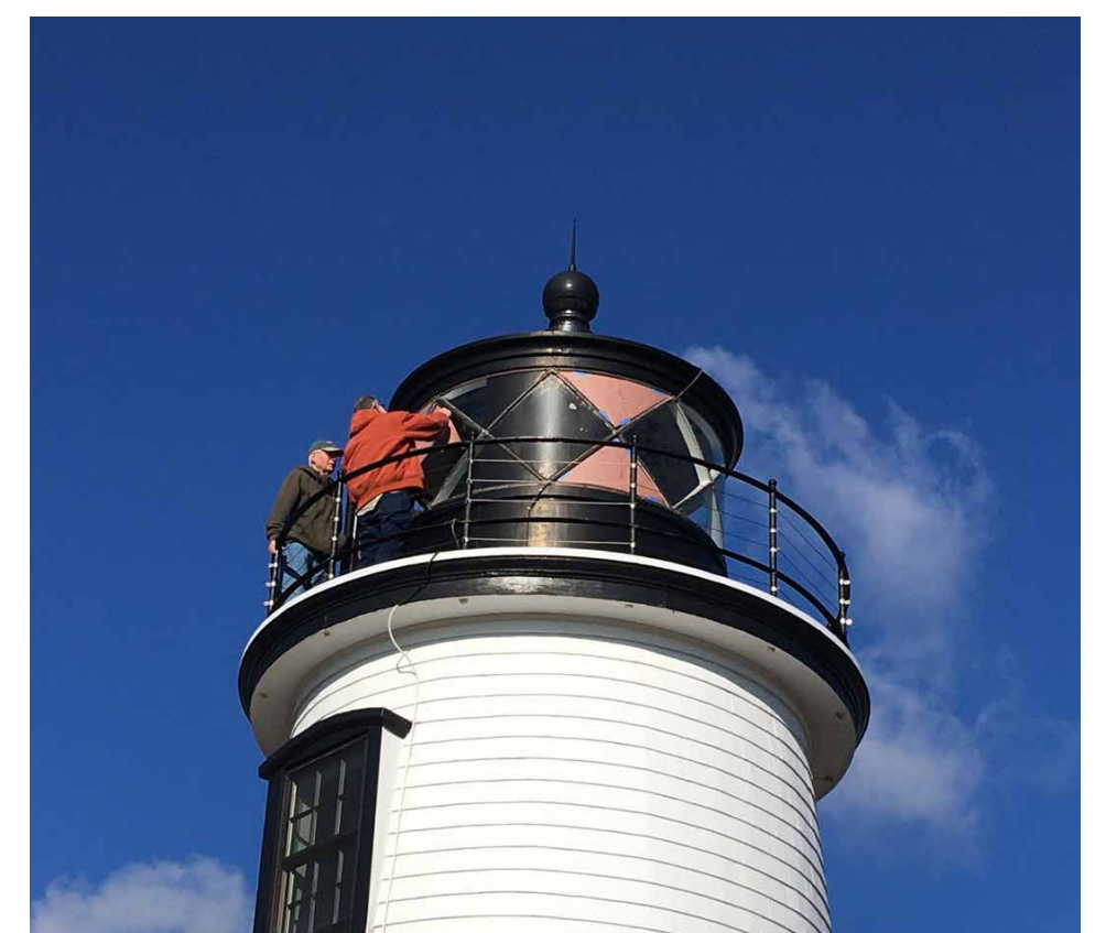
Installation of replacement glass
