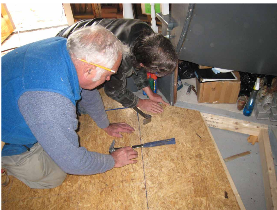
Replacement of lighthouse floor
